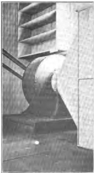
FIG. 50.—Exhaust fan showing connection of fan to tunnel.
