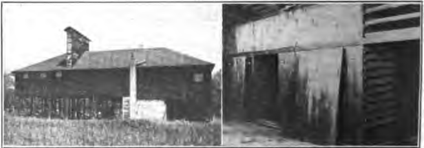
Figure 179. Views of Oregon Tunnel Evaporator on Abshire place near Geyersville. Lower ends of tunnels are shown in view on right. Used successfully in 1918 for prunes.
